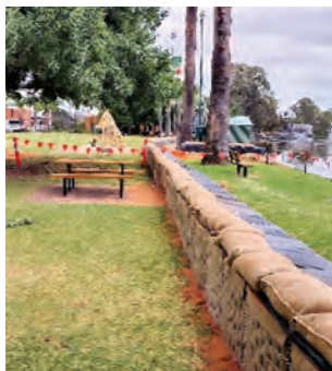
One of many effective flood banks created quickly throughout the district.
